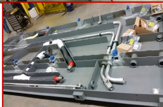
Skid Support-Integrated Piping
