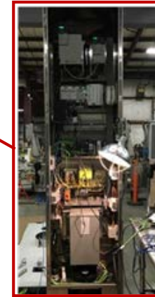
Process Control System (PCS)
